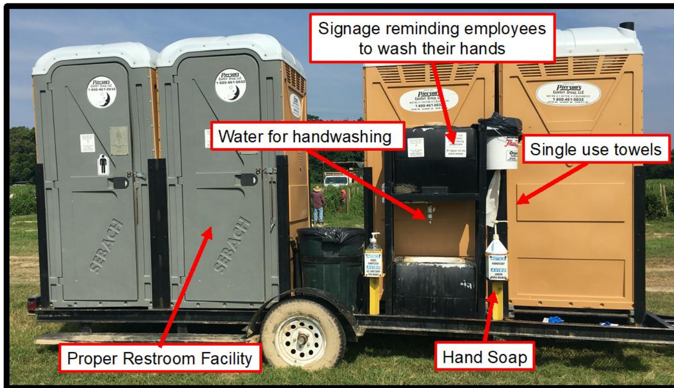
Figure 3. Clean restroom facilities, water for handwashing, hand soap, and single use towels must be available for employees and located near working areas that are easily accessible.
