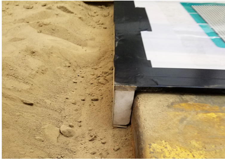
Figure D.3: 2" X 4" have been used as a peg to secure the wooden platform in place.
