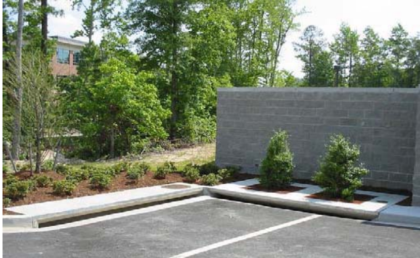
Figure 1. Filterra™ advanced bioretention system installation.
