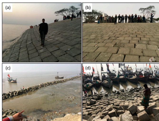
Figure 1. Revetments in Ramgati Upazila: (a,b) at Char Alexander, constructed 2015–2017; (c,d) at Ramgati Ghat, construction started in 2018 and ongoing at time of photos taken in January 2018 (photos by T. Crawford).
