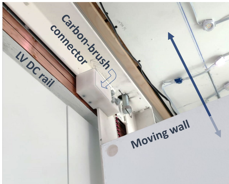
Figure 2: DC-powered moving wall (flex space)
