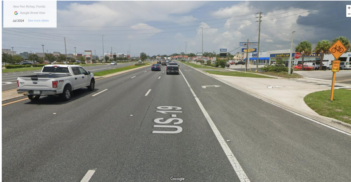
Figure 9: Northbound US 19 past Marine Parkway (Streetview)
