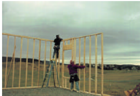
Fig 25: wall is raised into position
