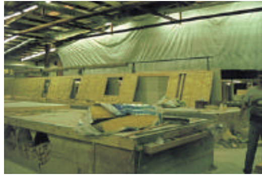
Fig 41: Pre-cut wood stored below
