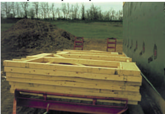
Fig 27: Pre-assembled wall panels
