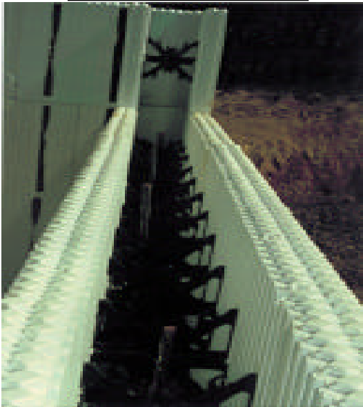
Fig 30: Reinforcement in forms
