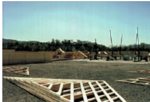
Fig 52: Trusses are stacked in yard
