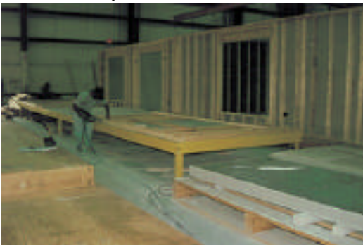
Fig 40: Wall construction, on table
