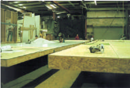
Fig 38: Sanding the Sub-Flooring
