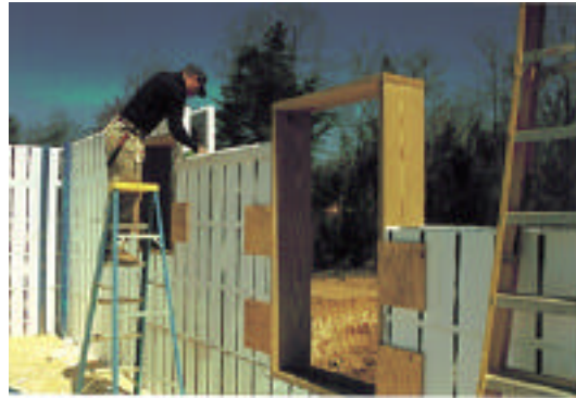
Fig 29: Forms are assembled
