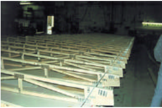
Fig 46: Trusses assembled to form roof
