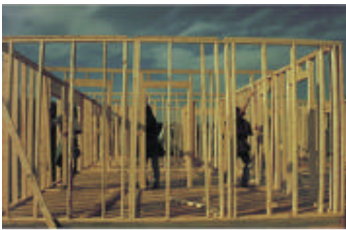
Fig 36: Wall assembly is lifted in place
