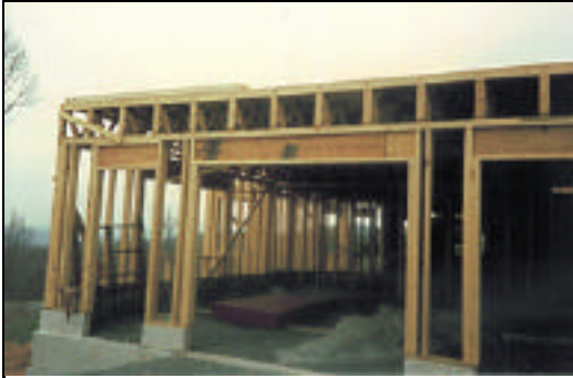
Fig 32: Floor trusses
