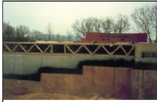
Fig 33: Floor Trusses
