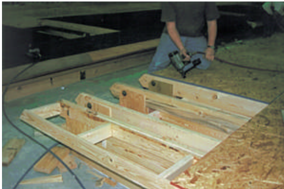
Fig 48: Hinged roof with knee wall below
