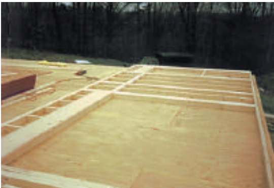
Fig 24: wall framed flat on subflooring
