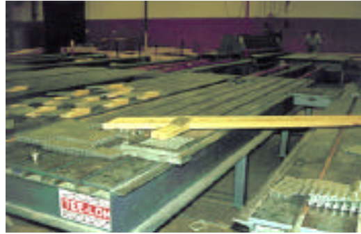
Fig 50: Truss assembled on table
