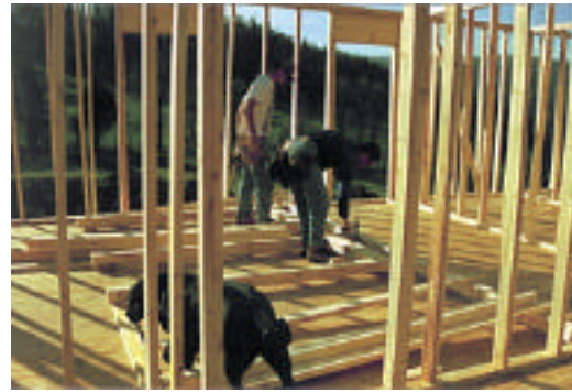
Fig 35: studs are attached to top
