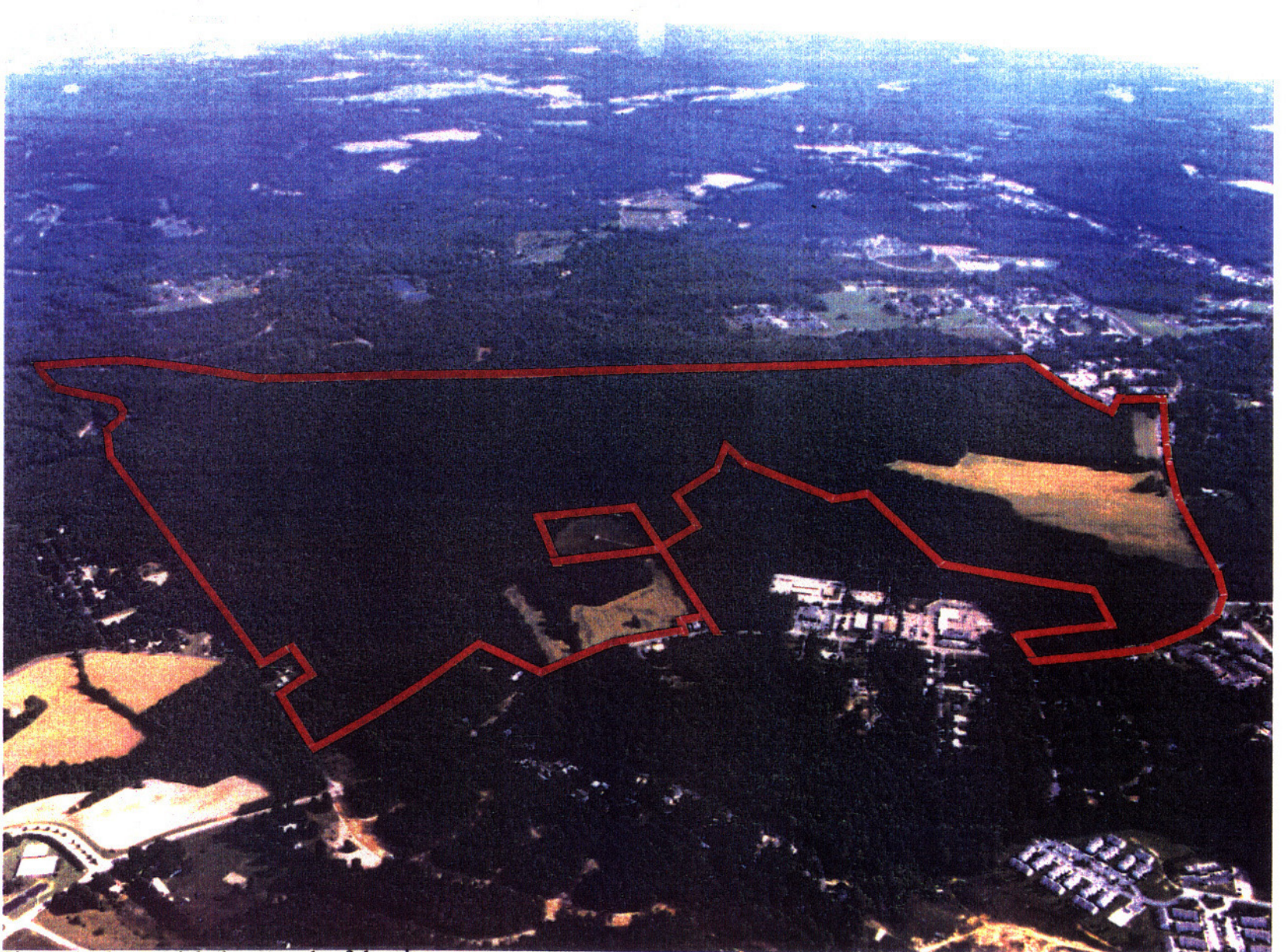
Figure 4.16 Aerial photograph of the site
