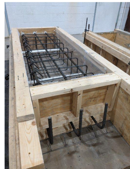
Figure 3-3 : Precast Construction
