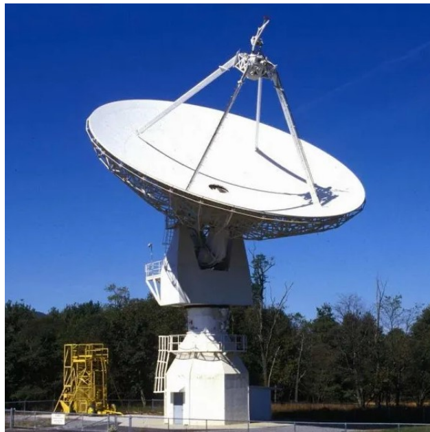
Figure 1.1: The Green Bank 20-Meter Telescope, an example of a focus-fed axisymmetric paraboloidal reflector antenna. Picture is sourced from [3].
