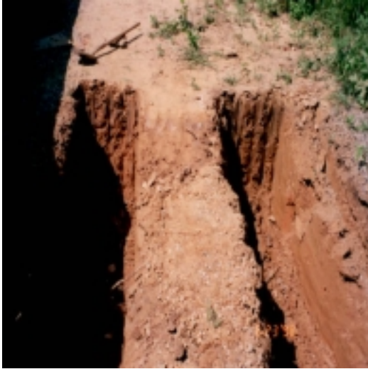
(a) Parallel trenches for digging block samples.
