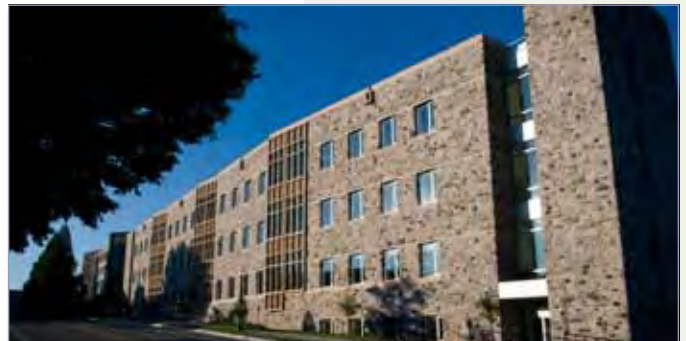
Side View of the Newest ICTAS Building
