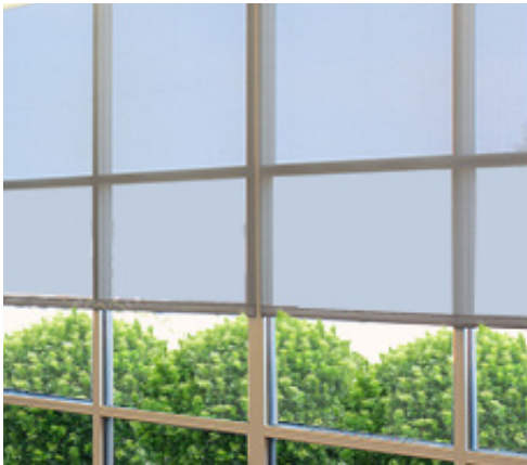
Adjustable Window Covering Glare can come from a direct beam of sunlight, its reflections, or from the window itself, even when no direct sunlight enters. When it is brighter outside the window than inside the classroom, the window can be a potential glare source. Window coverings can be used to reduce this
