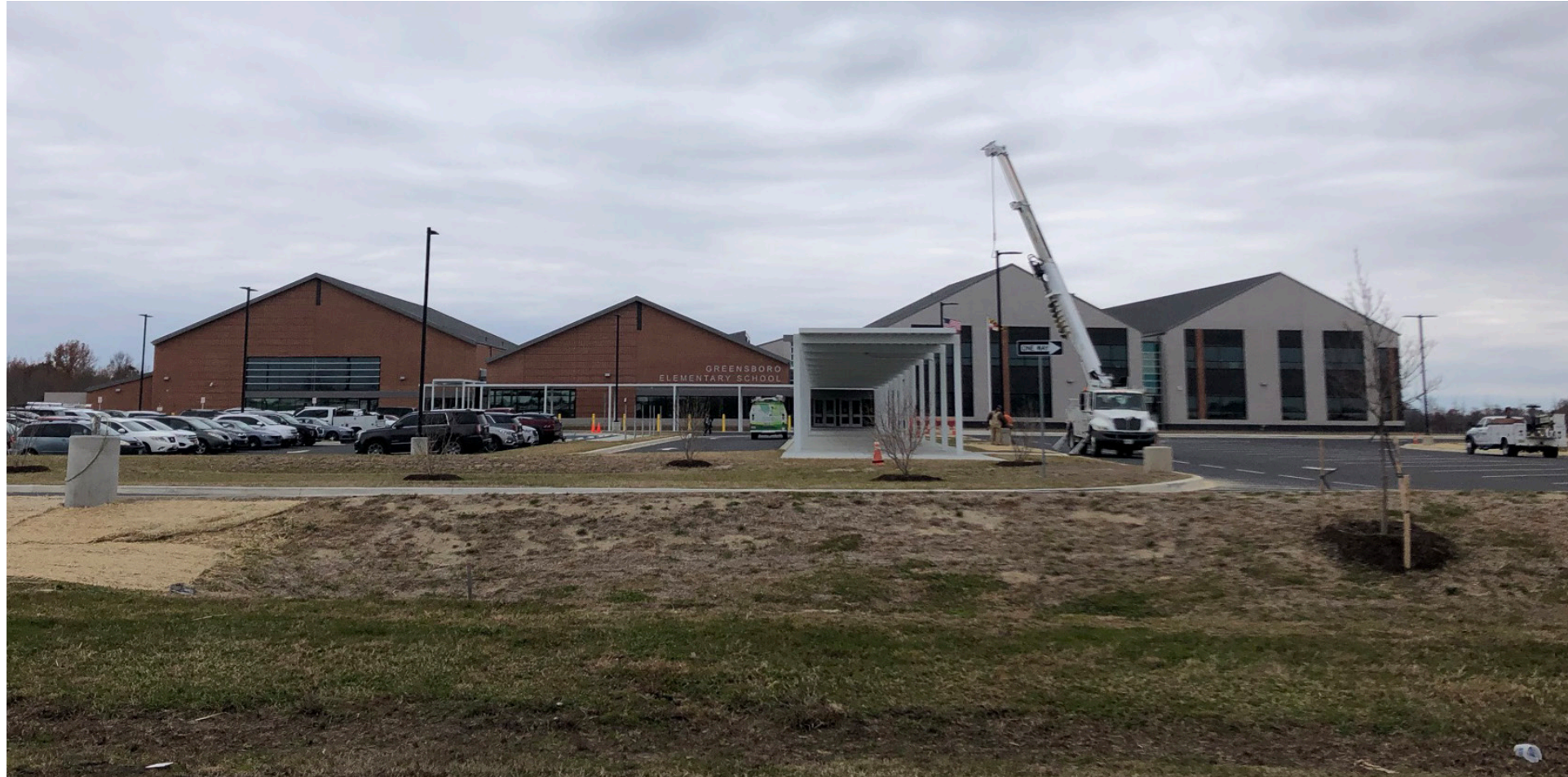
Greensboro Elementary School on the selected site.
