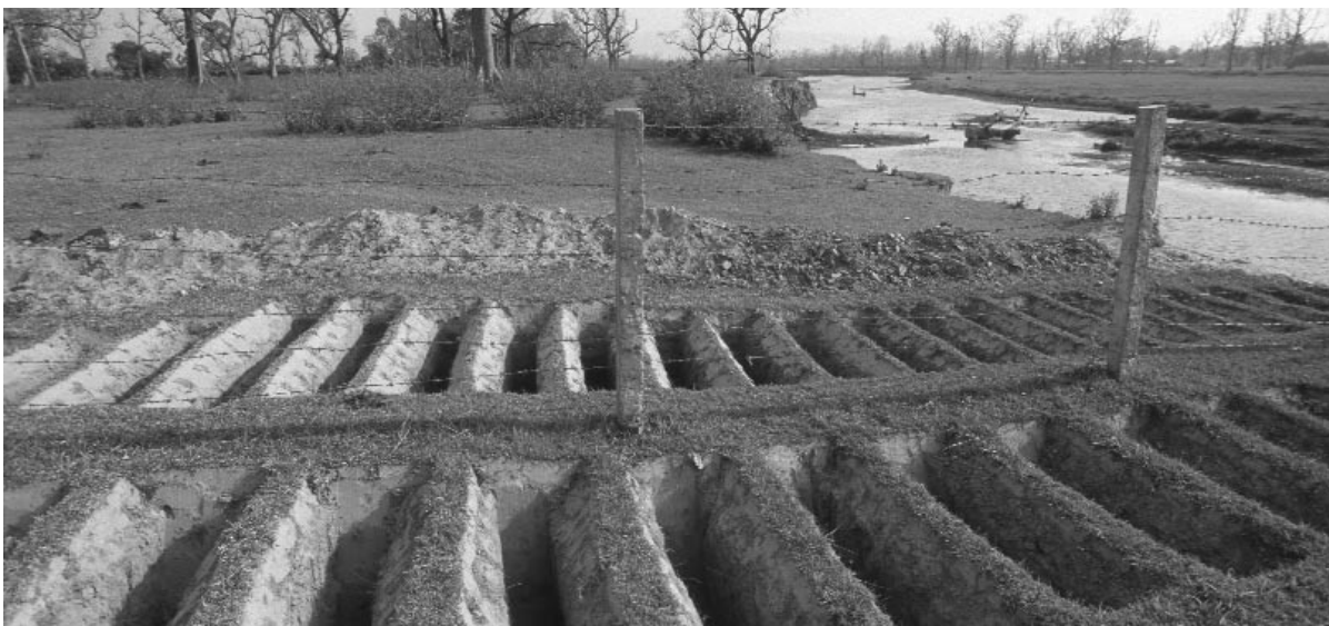
Ditches dug on both sides of a fence in order to keep rhinos away, so that they do not damage the fence. Village area on the outskirts of Royal Chitwan National Park, Nepal.
